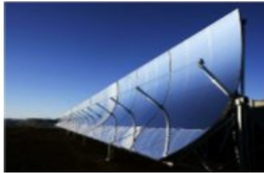
Figure 1.3: Parabolic trough collector
