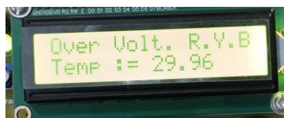
Figure 3. Over voltage fault detection on LCD display
