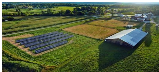
Figure 1-.Farm-type photovoltaic-power-generation system.
